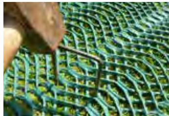
Fix using steel u-pins
