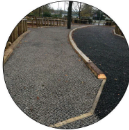
Backfilled with gravel
